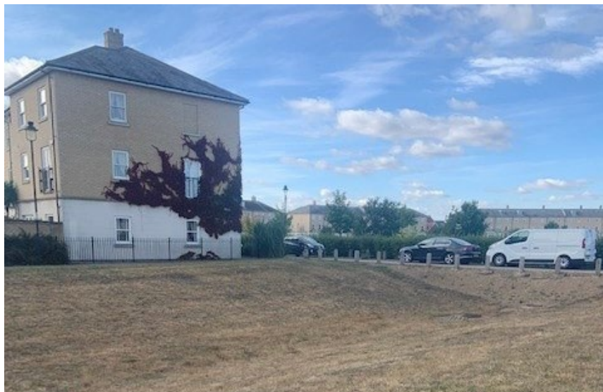
Figure 3 Infiltration basin at Ravenswood, Ipswich.
