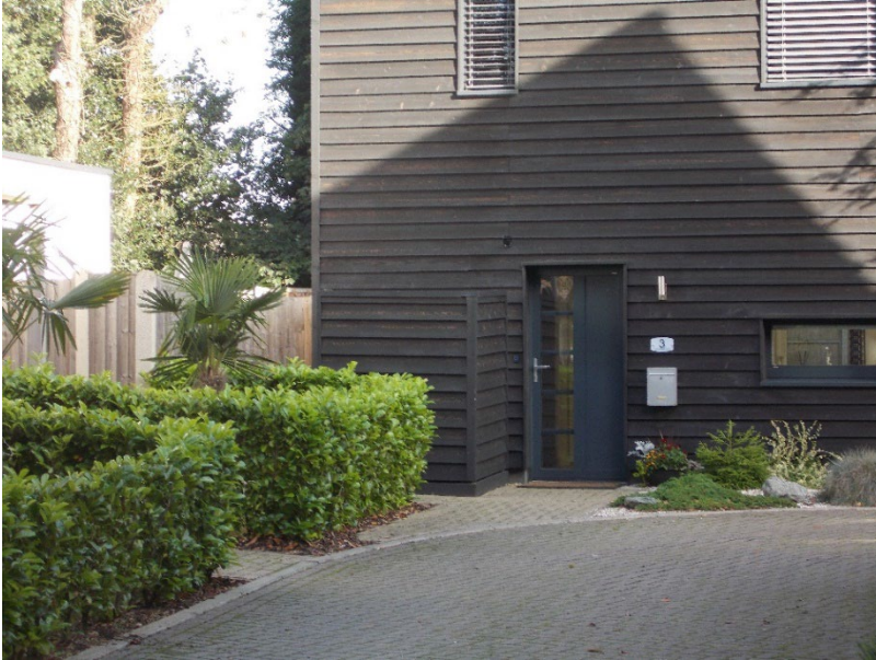
Figure 12 Wheelie bin storage screen by front door constructed from the same black horizontal timber as the house
