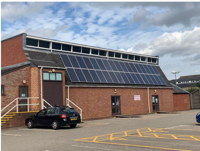
Figure 19 Solar panels in Woodbridge
